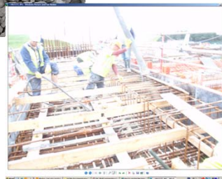
Casting GGBS Concrete at Sellafield
