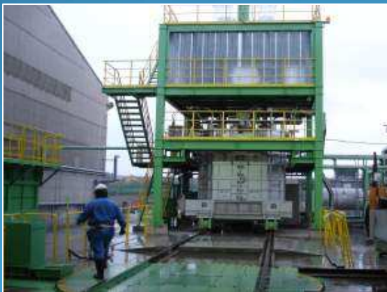
Rail Mounted Box at Melt Station
