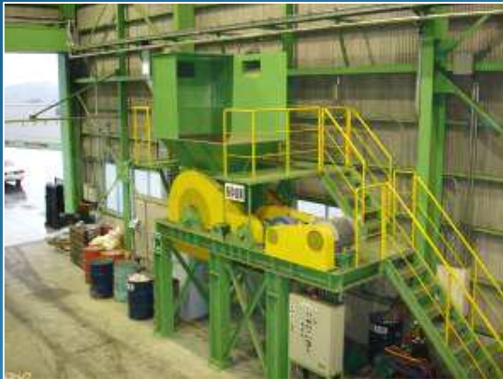
Crusher for Concrete & Debris
