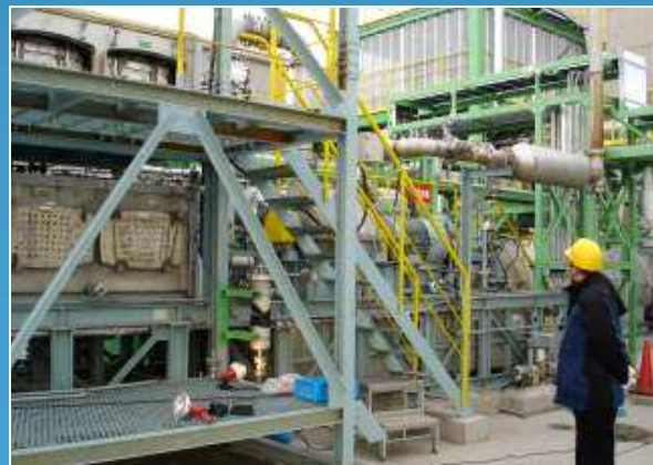
Off-Gas Treatment Equipment
