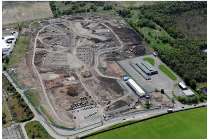
View of the former HMP Low Moss after demolition.
